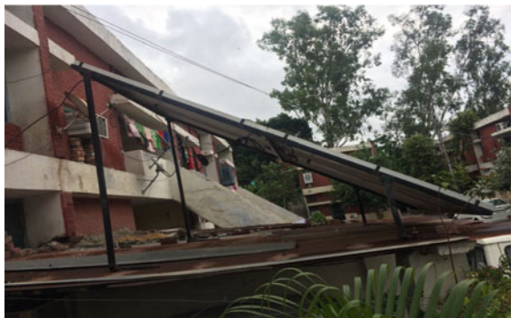
Fig. 5 Solar panels mounted at optimum angle
