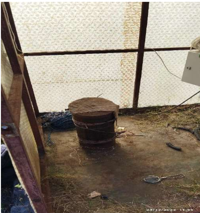
Groundwater monitoring station at Gopeshwar.
