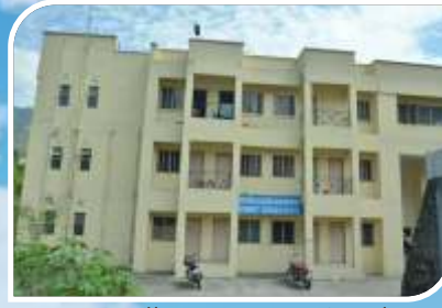
Aryabhata Research Boys' Hostel, Chauras Campus
