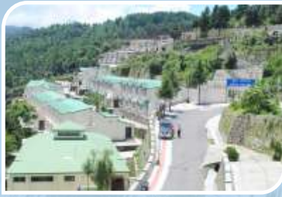
Boys' Hostel, Tehri Campus
