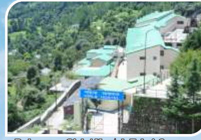
Balganga Girls' Hostel, Tehri Campus
