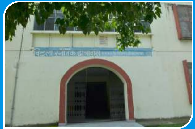
Chaukhamba U.G. Boys' Hostel, Srinagar Campus
